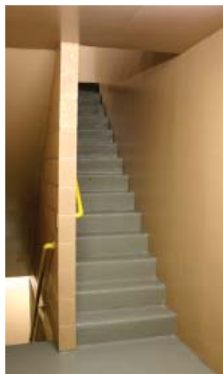
Distribution at high angles allows light to reach the top stair
