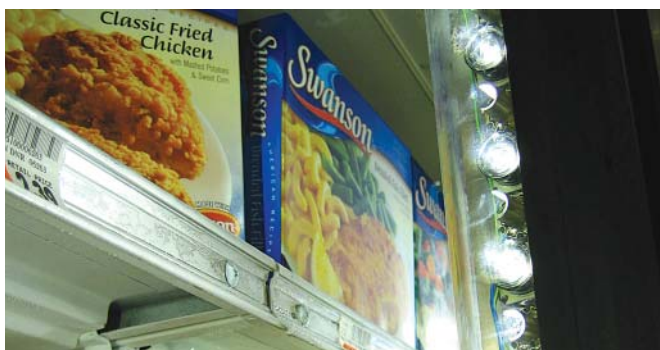
White LEDs were mounted vertically and aimed to graze the front of the shelves.
